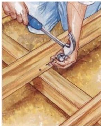
Secure the floor frame to the foundation skids with angles (outside skids) and toenails (center skid).
