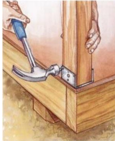
Anchor the six posts to the floor with metal post bases. Use galvanized nails to fasten the bases and posts.
