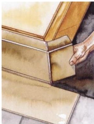
Cut the horizontal flanges of the bottom piece of skylight flashing and wrap the ends around the frame sides.
