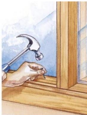
Attach the outer window stops, with the beveled stop at the bottom. Nail the center stops to the mullion.
