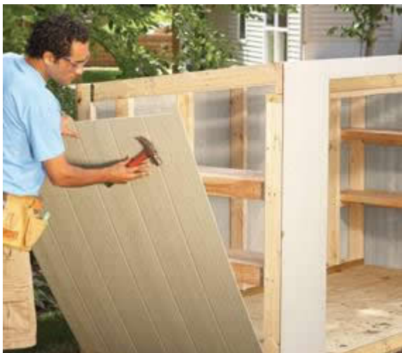
PHOTO 6: INSTALL THE SIDING
