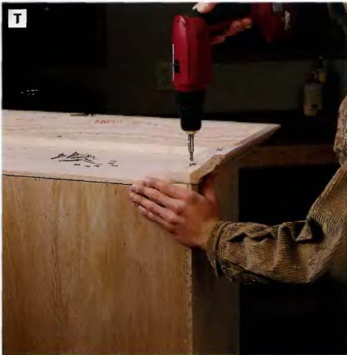
PHOTO T: Attach the crown frame to the top of the cabinet with screws and washers. The screw slots in the tops of the scrap wood backer frame allow for cross-grain expansion and contraction of the solid wood top.
