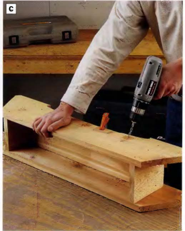
PHOTO C: Fasten the planter sides to the ends and bottom with nails, then drill three angled \frac{1}{4} -in.-dia. weep holes through the side where the bottom of the planter slopes to its lowest point.
