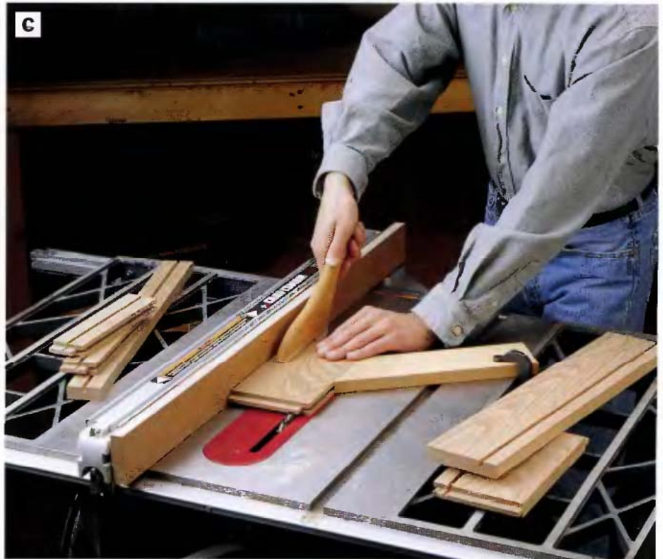
PHOTO C: Cut \frac{1}{4} \times \frac{3}{8} -in. grooves for the upper and lower chest bottoms into the side and front rails. Use a featherboard and pushstick.
