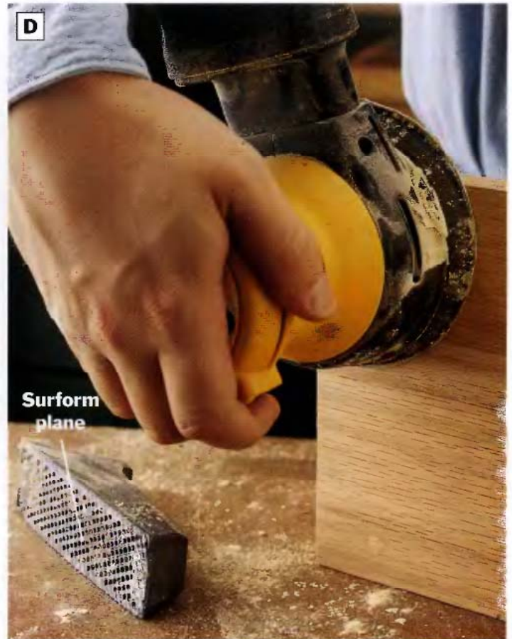
PHOTO D: Shave the plugs so they're nearly flush with the surrounding wood surface using a Surform plane or a wood rasp. Sand away the remaining waste with coarse sandpaper.
