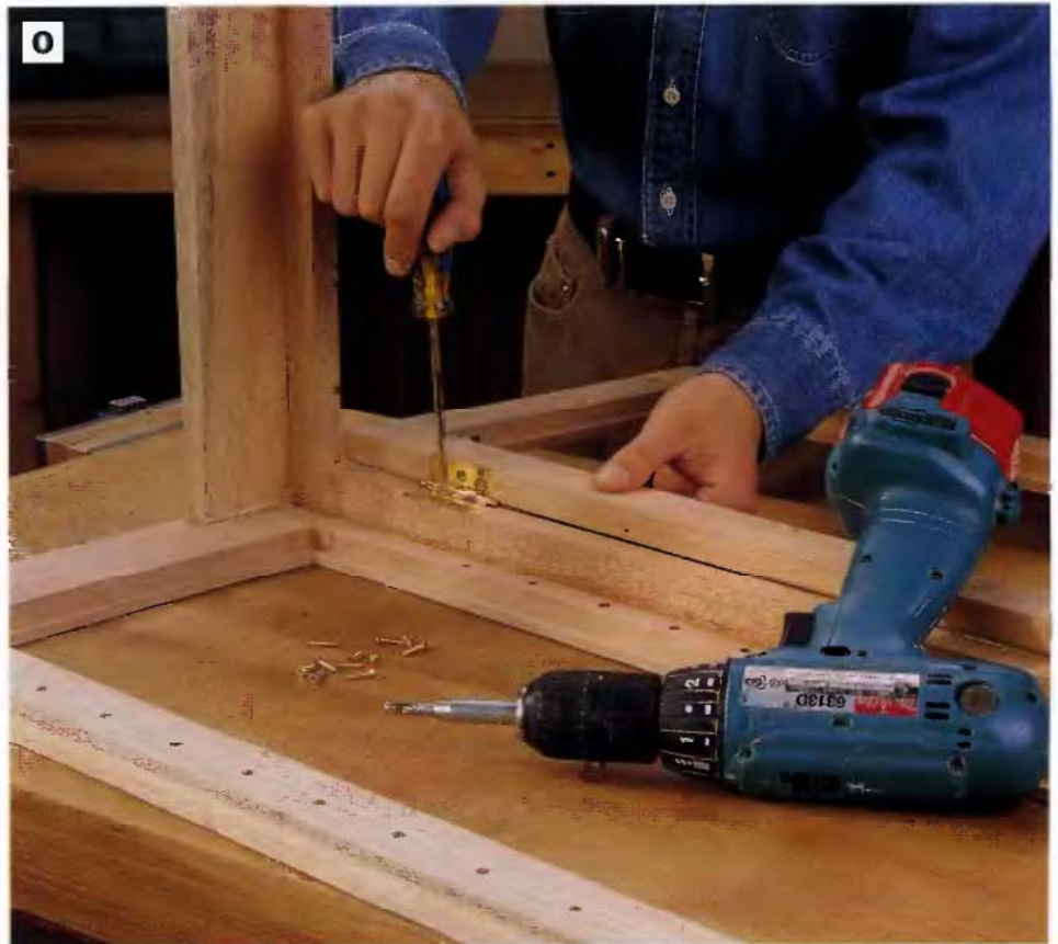
PHOTO O: Cut hinge mortises into the edge of the face frame stile and attach the door to the cabinet with hinges and screws. Drill pilot holes for the screws to keep them from splitting the wood. Support the door from beneath as you attach the hinges.
