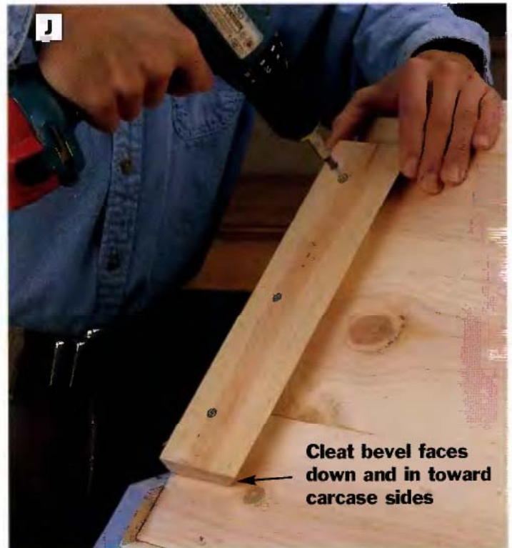
PHOTO J: Attach French cleats to the sides of the cabinet, flush with the top of the carcass. The cleat bevels face down and into the sides.
