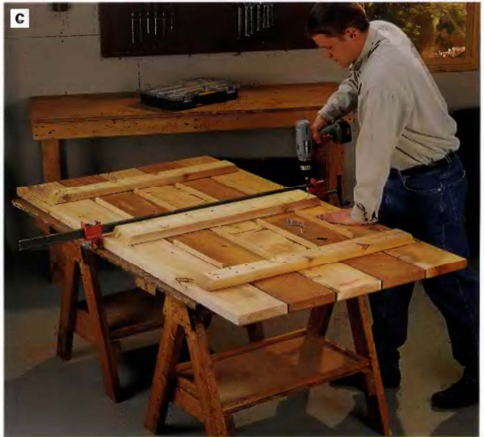
PHOTO C: Mark locations for the three table stretchers on the bottom of the tabletop, then fasten the stretchers to the table slats with 2½-in. galvanized deck screws. Set ¼-in. spacers between the slats before you fasten the stretchers to keep the slats held evenly apart.
