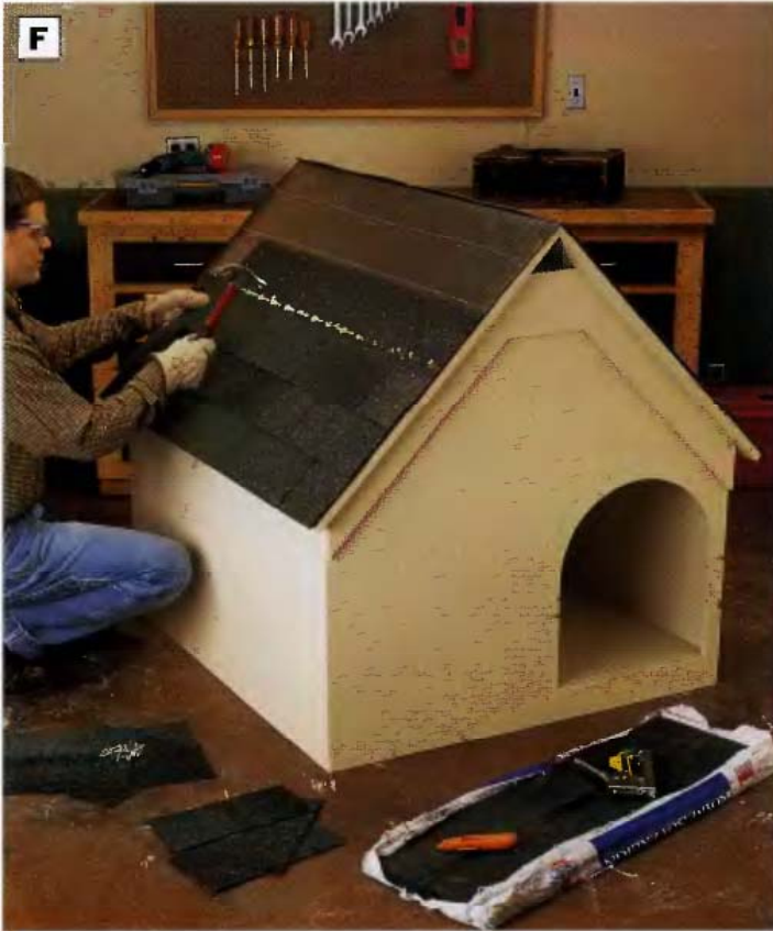
PHOTO F: Staple a layer of building paper over the roof panels, then shingle the roof, starting from the bottom and working up to the peak.
