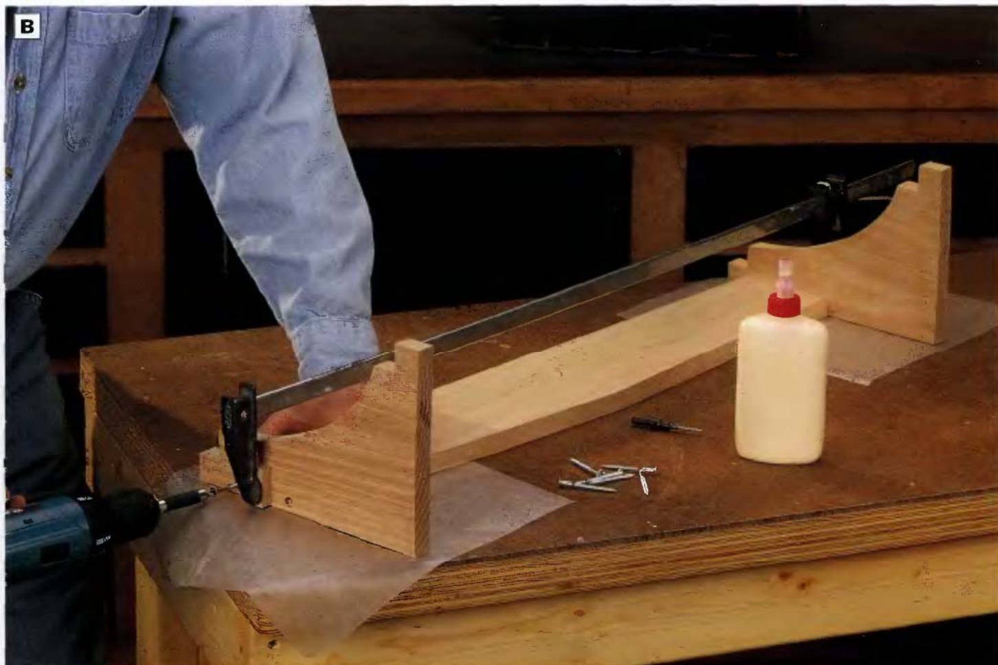
PHOTO B: Fasten the coatrack ends to the back with glue and flathead wood screws driven into counterbored pilot holes. Clamp the parts together first to hold them securely while you install the screws.
