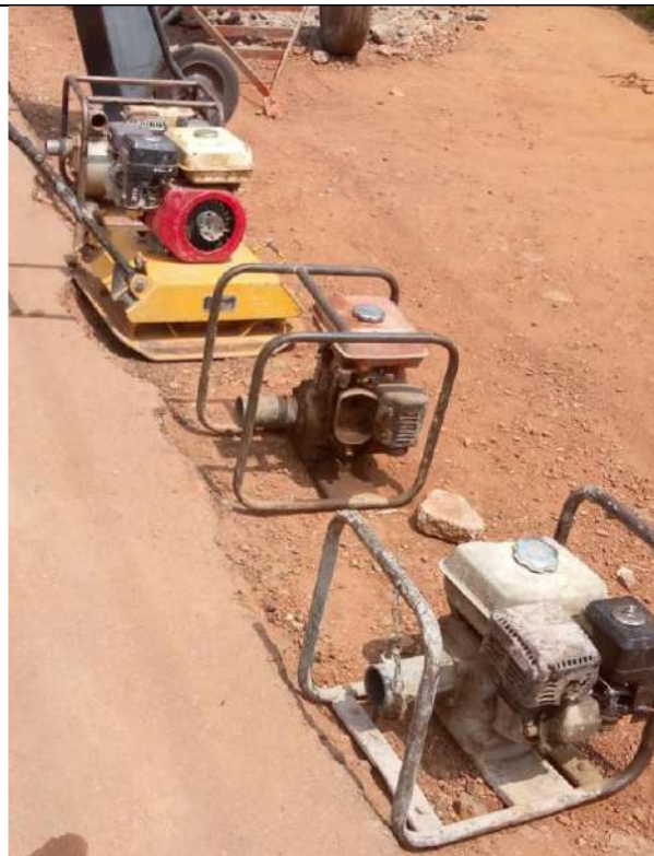
WATER PUMPS & COMPACTOR EXCAVATOR CAT
