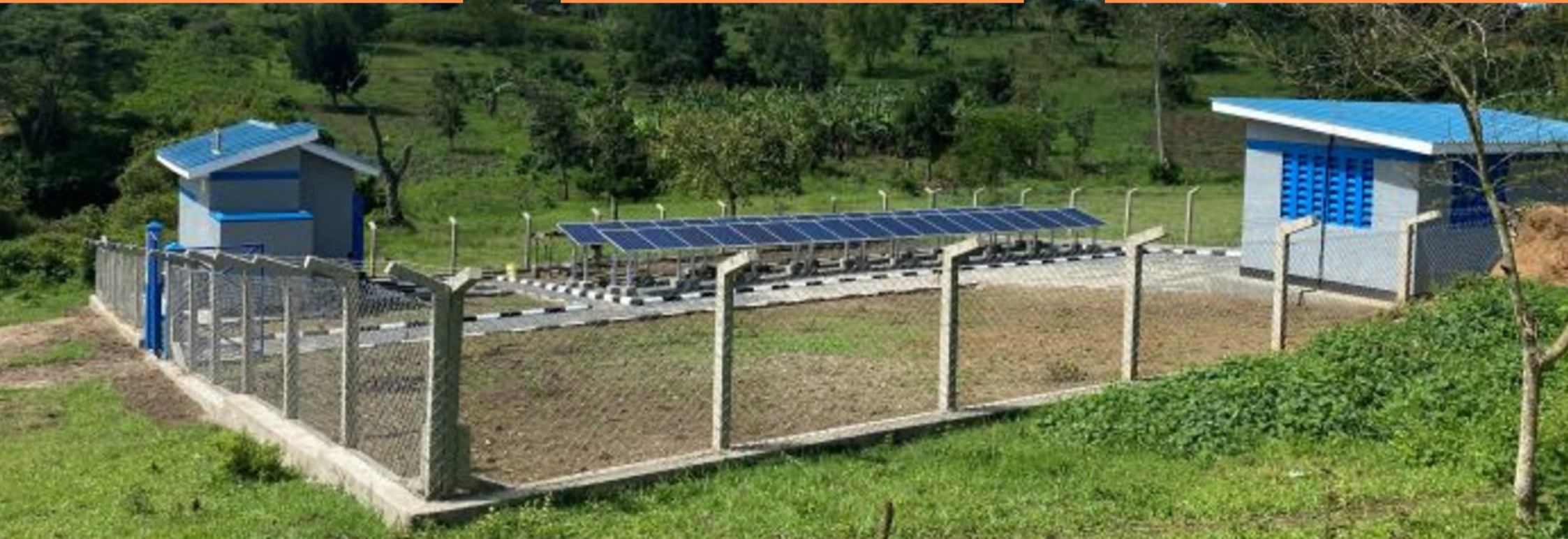
CONSTRUCTION OF SOLAR POWERED WATER SYSTEM IN RHINO CAMP REFUGEE SETTLEMENT- MADI OKOLLO DISTRICT. (REF- UG/ONL-WCP-KFW-01/09/21) UNDER OXFAM
