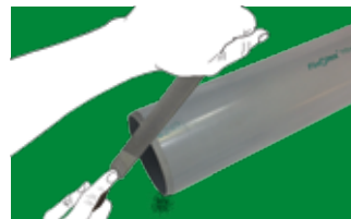
4. Chamfering & Cleaning
