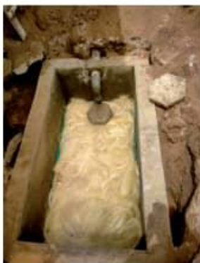
Etape 9: Installation de filasse
