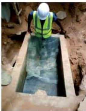
Etape 7: Installation des grillages
